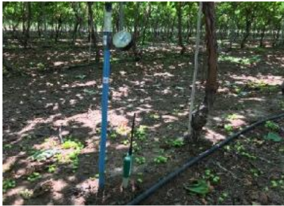
Wireless moisture probes with analog redundancy, Israel
