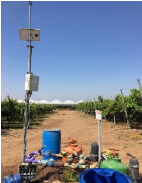
Wireless irrigation controller, Israel
