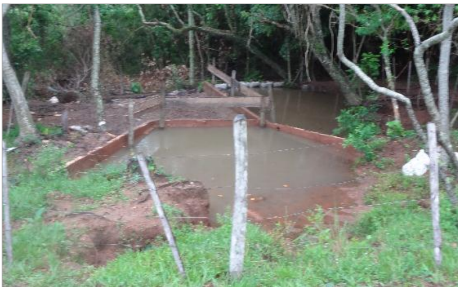
A natural spring in Paraguay fenced off to prevent cattle entering the water and damaging the banks. The cattle can reach through the wooden rails to drink from the pool formed with reclaimed house bricks
