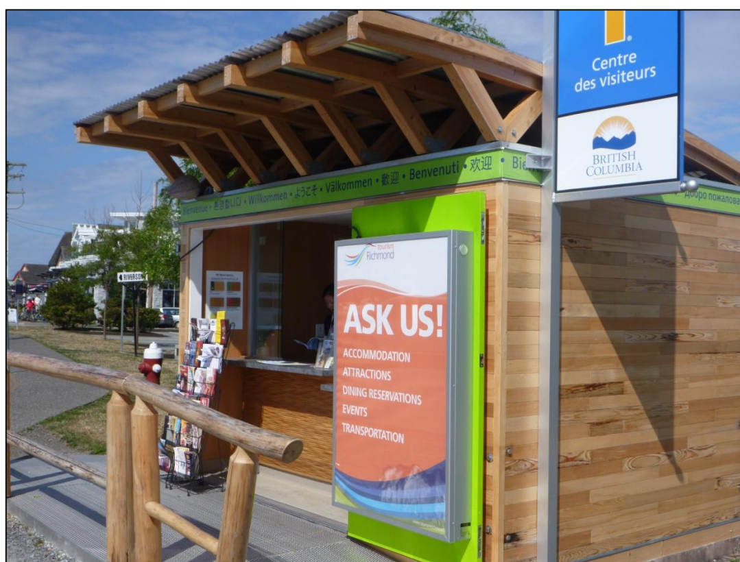
Tourist information booth in Vancouver using unfinished small dimension glue-laminated roof structure and timber cladding
