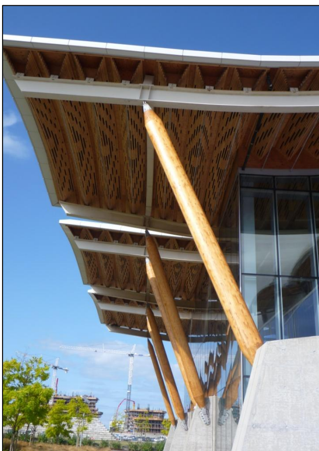
Richmond Oval Olympic ice-rink using dead Pine in panels produced by Structure Craft to promote the properties of the large volumes of dead timber available.
