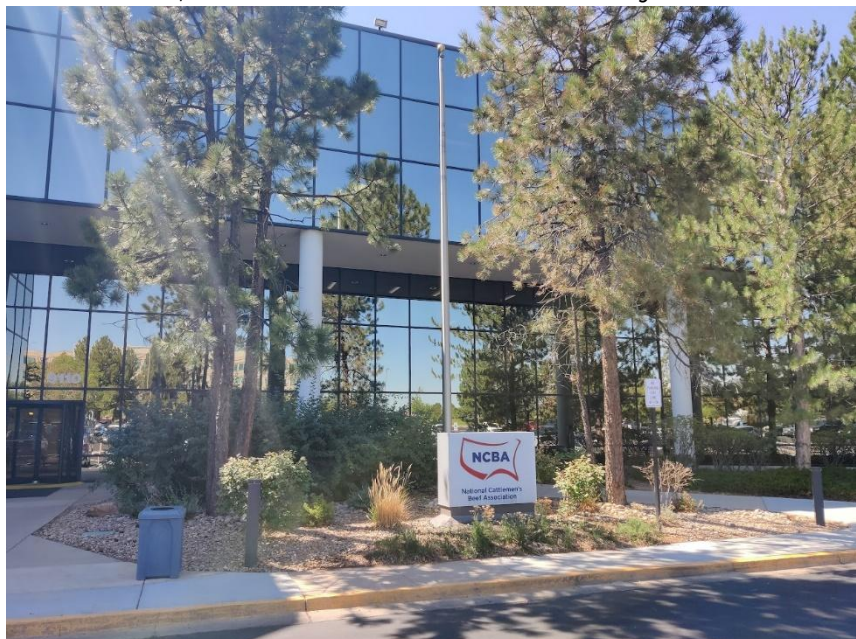
Figure 23: NCBA offices Denver Photo: Author's own.
