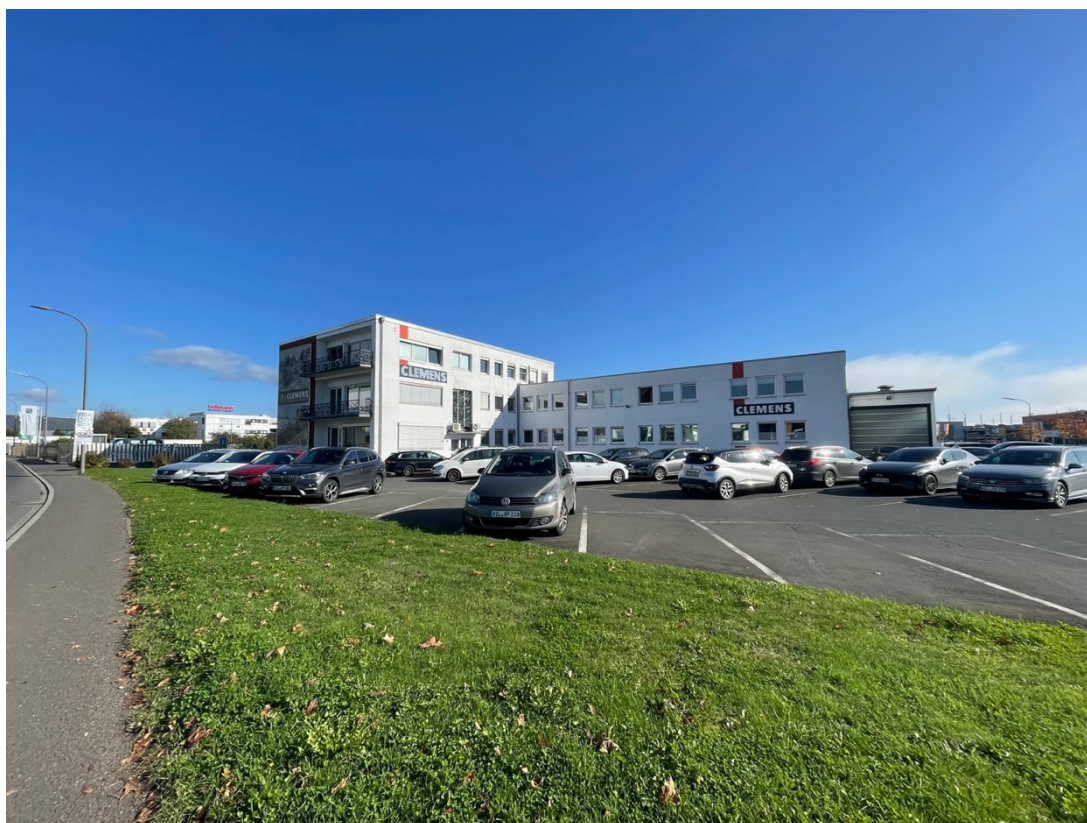
Figure 6 Head Office of Clemens Technologies in Wittlich, Germany
