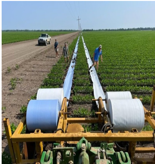
Figure 15 : Mechanical installation of Polypipe (Source: author, Mer Rouge, Louisiana , USA, 2023)
