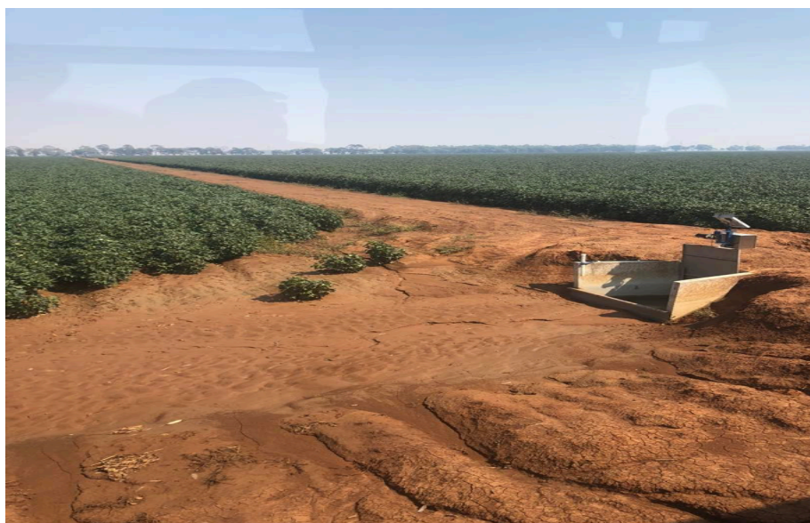
Figure 8: Bank-less check for controlling flow of water between bays (Source: author, Griffith, NSW 2020).
