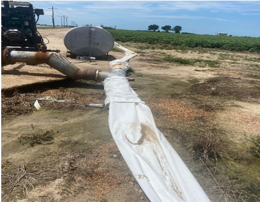
Figure 14: Polypipe connected directly to a bore (Source; author, Mer Rouge, Louisiana , USA, 2023)
