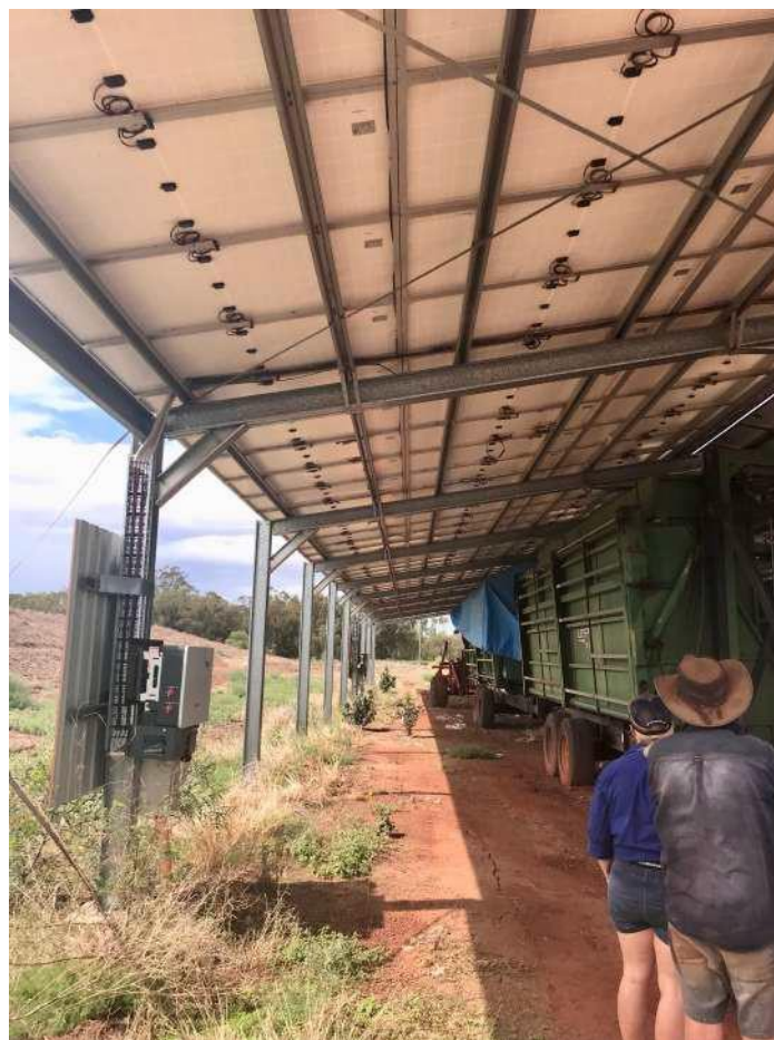
Figure 20: Solar roof, Australia; Authors Own
