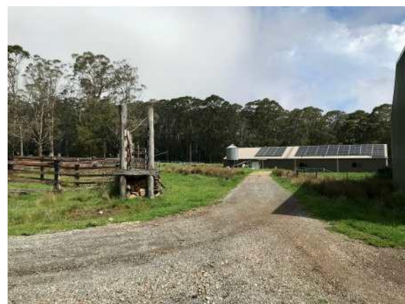
Figure 15: Pecora dairy rooftop solar; Authors own
