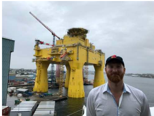
Figure 7: 900MW transmission platform Haugesund, Norway; Authors own
