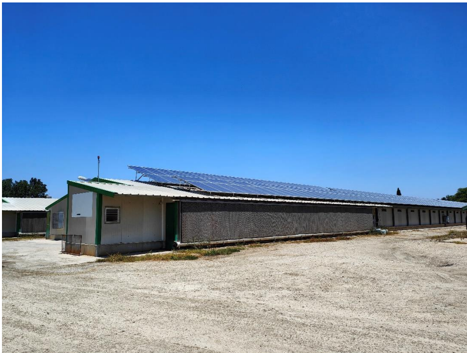
Figure 6. Broiler shed with cooling pads in Israel
