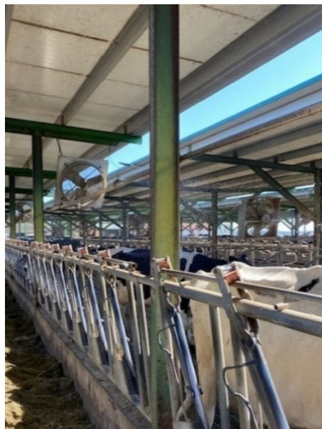
Figure 18 - Dairy farm in Castilla la Mancha, Spain. Fans with misters (Source: Author, 2023).
