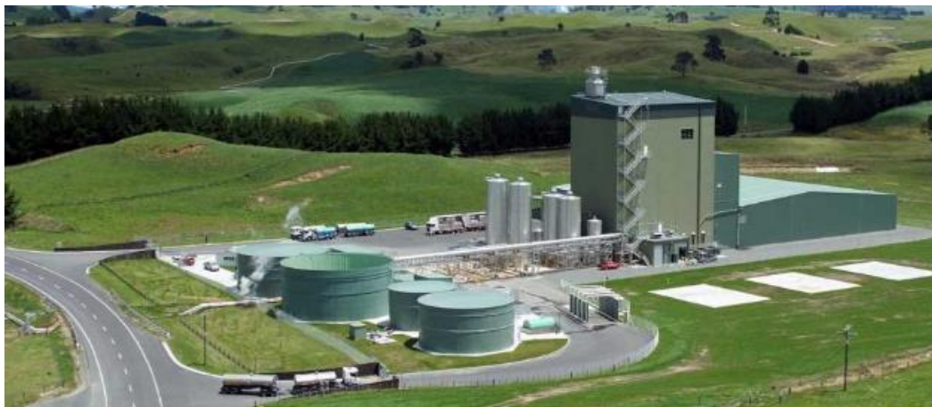
Figure 49: Miraka's greenfield milk drying facility in Waikato, NZ, was commissioned in 2011. Source: Tuasopaki.com
